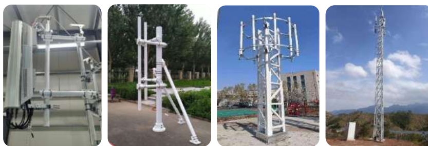
a) Antena Pole b) Roof Pole c) Rooftop Tower d) Greenfield Tower.
